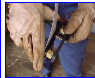
Employee removing BHISD and connecting a torch.
